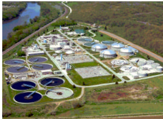
Cedar Rapids water pollution control system.
