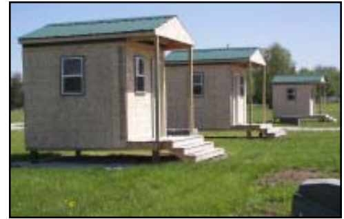
Safe City's structures continue to take shape on IAMU's Safety & Training Field. Work on the six small buildings will continue this summer.
