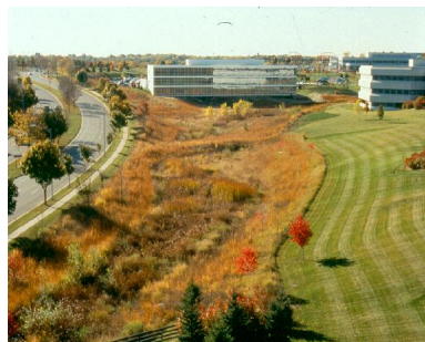
Well-vegetated bioswale after installation (CDF Inc.)
