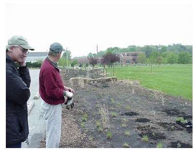
Bioswale under construction in Davenport, Iowa (River Action)
