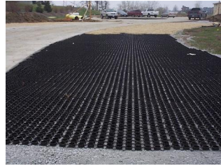
Porous pavement installations, Iowa City, Iowa.
