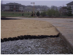
Porous pavement installations, Iowa City, Iowa.
