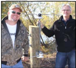
A new fence on IAMU's property simulates electric poles and lines. City of Ames electric personnel (top) and IAMU's Steve McLaughlin (bottom photo, left) and Tom Erickson were instrumental in erecting the unique fence.
